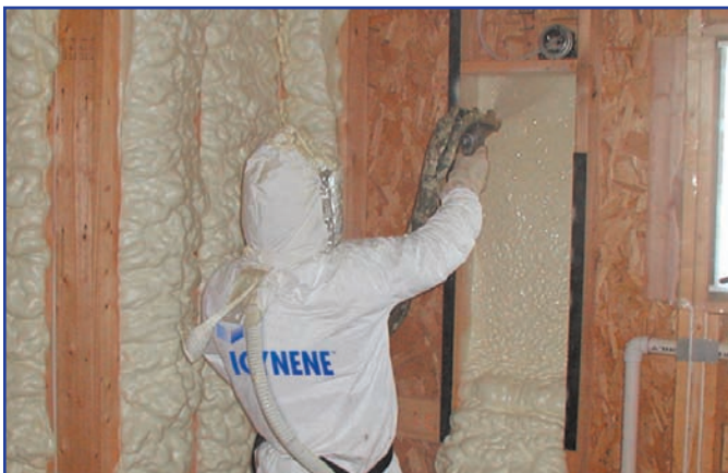
Icynene is sprayed directly into the exterior wall. The foam softly expands to fill all of the cracks and crevices. Any excess foam is easily trimmed in preparation for drywall.
