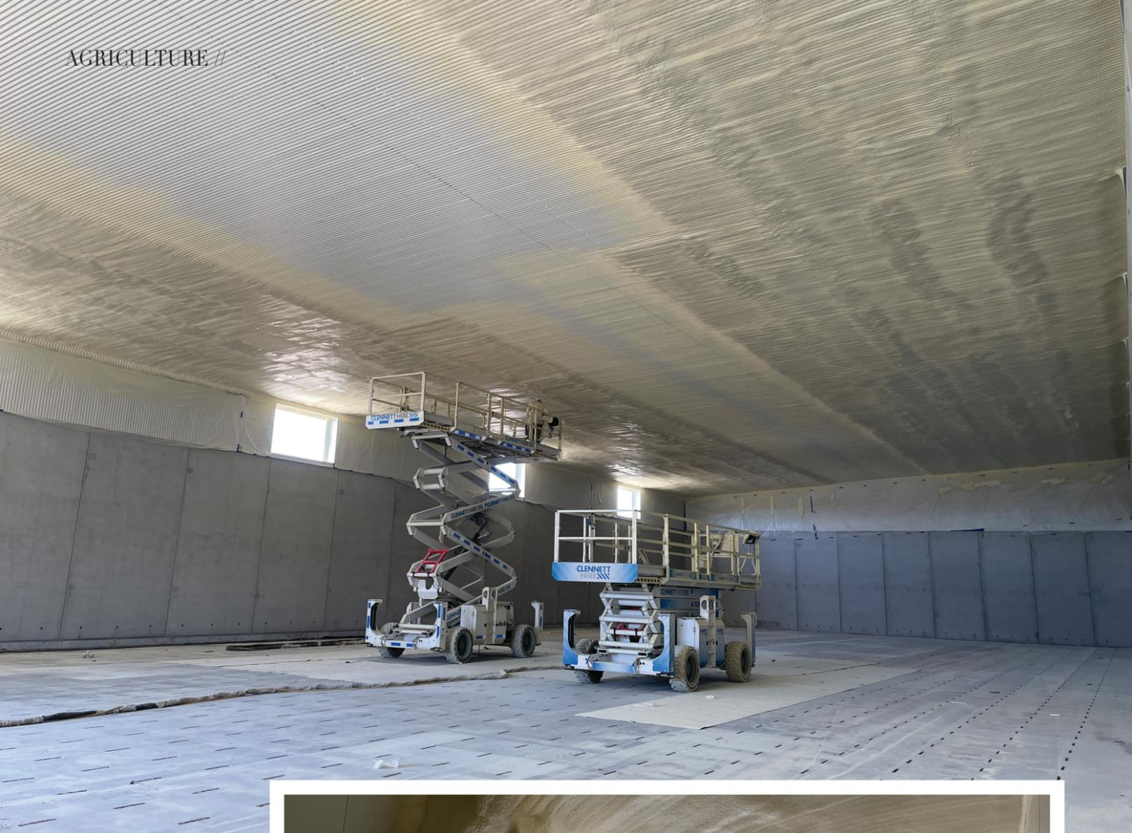
**ABOVE:** The sprayers apply a trail of RamBoard to the store's floor for the scissor lift to roll over while spraying the ceiling; **RIGHT:** A shot of the internal walls and upper hallways that connect the stores.
