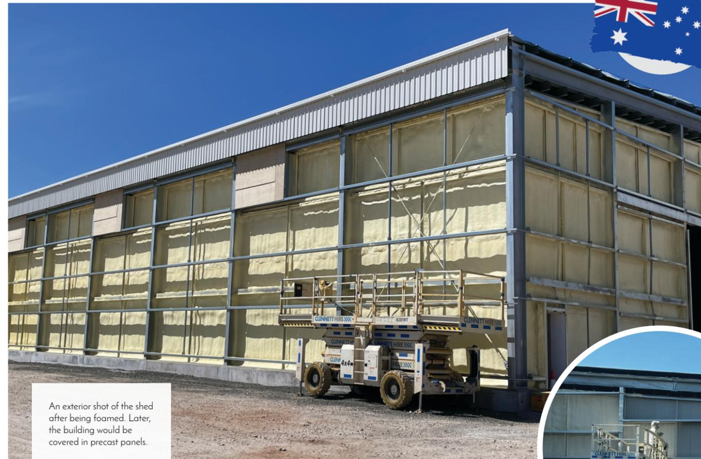
An exterior shot of the shed after being foamed. Later, the building would be covered in precast panels.
